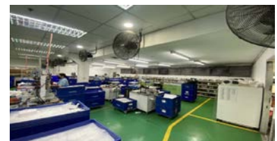
Replaced air conditioners with air-cooled chillers Janome Thailand, Co., Ltd.
